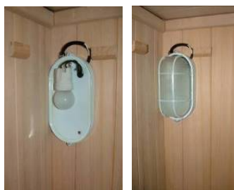
FIG-11 Assembling the light
