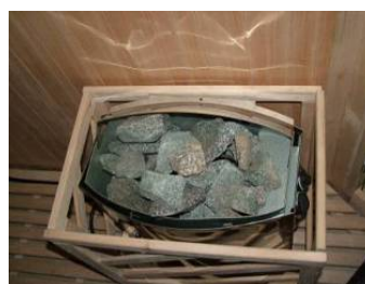
FIG-18 Place sauna stone
