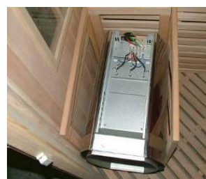
FIG-16 connect the power supply line of stove
